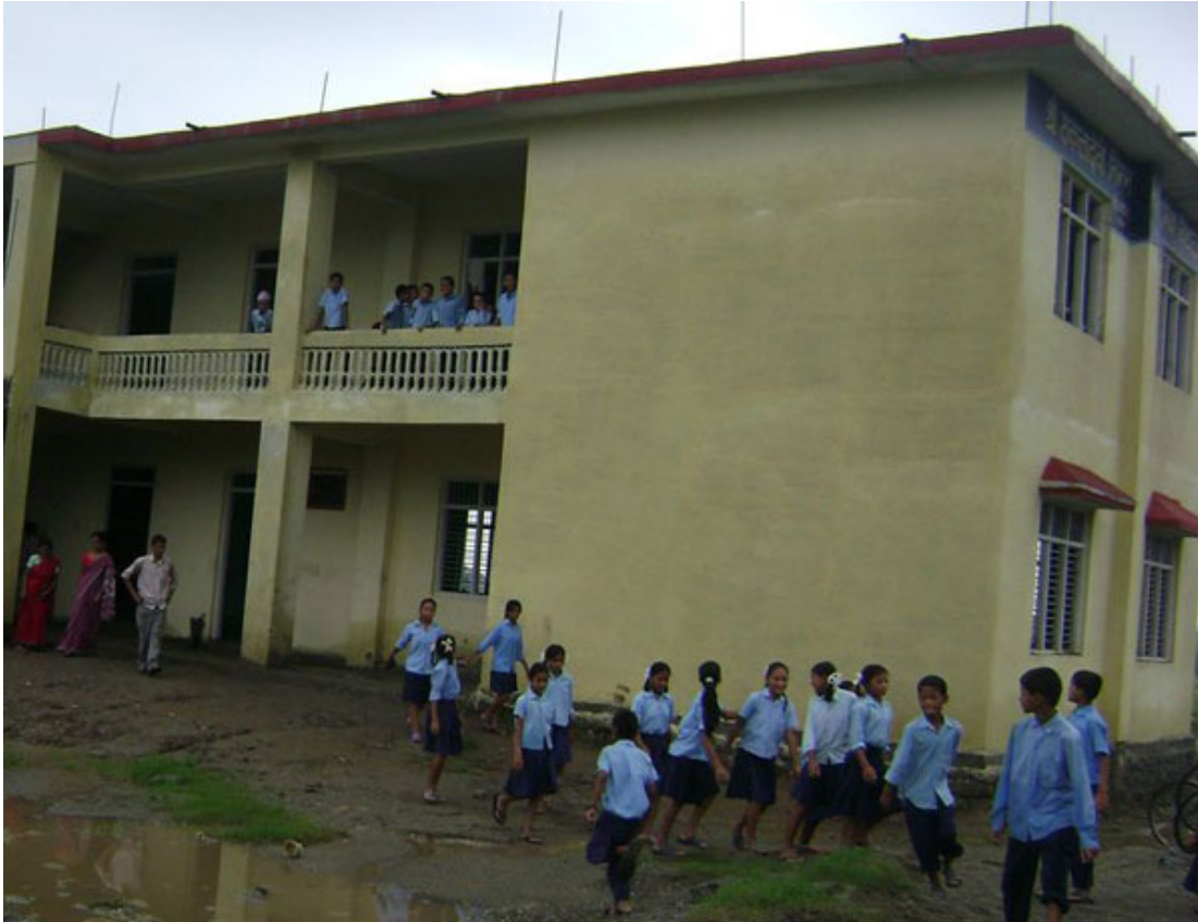
Newly constructed school building.
